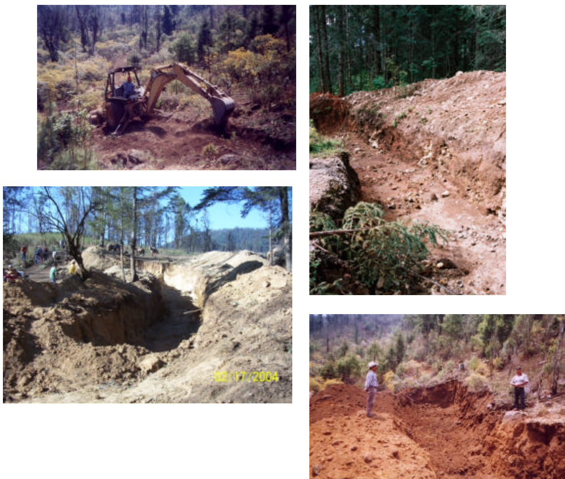
Figure 7. Examples of trenches built in the region to stop the illegal loggers (WWF pictures).
